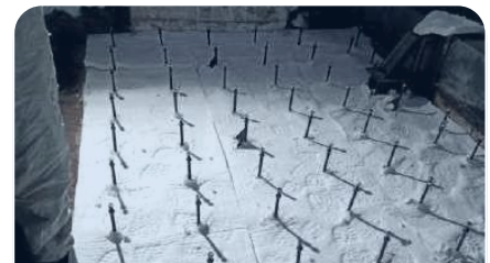
Casing and refractory repair
