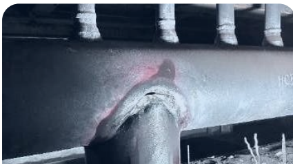
Diverter damper shaft replacement
