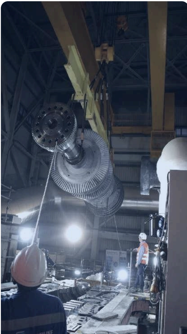
Steam turbine major overhaul
