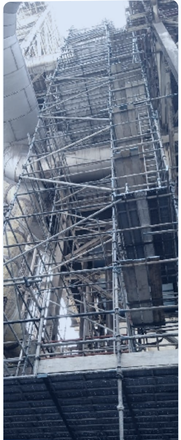
Boiler scaffolding during a shutdown
