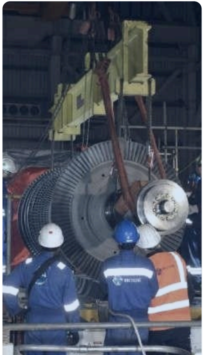
Steam turbine major overhaul
