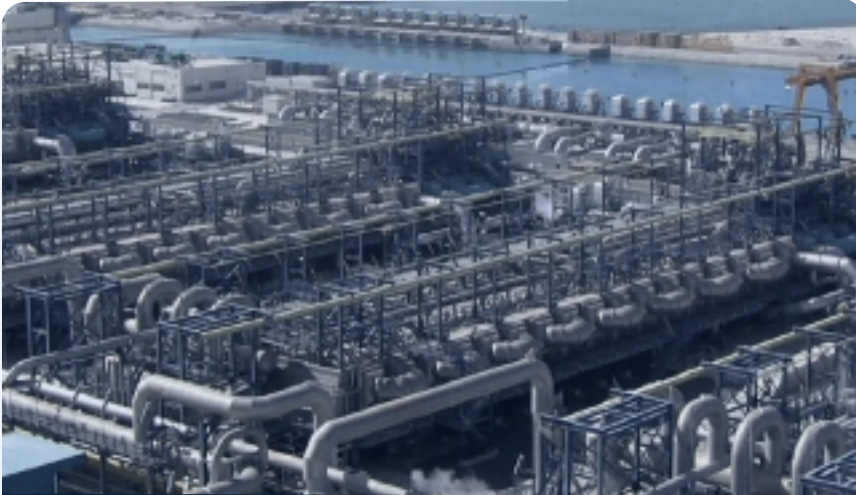
EPC project site, water and power plant
